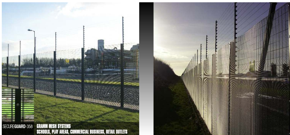
Figure 1: Indicative photos of the security fence.
